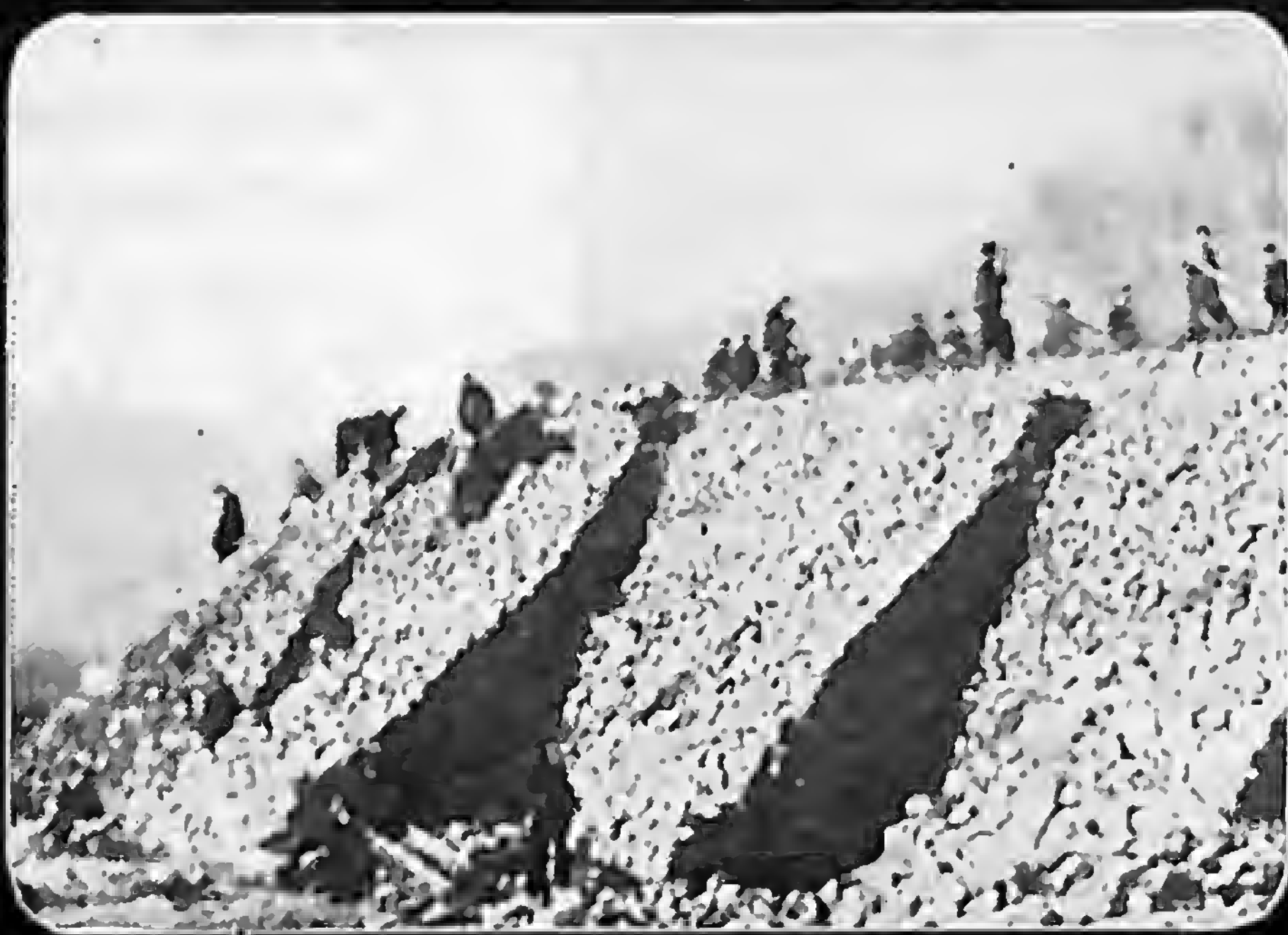
Making lime without a kiln.
